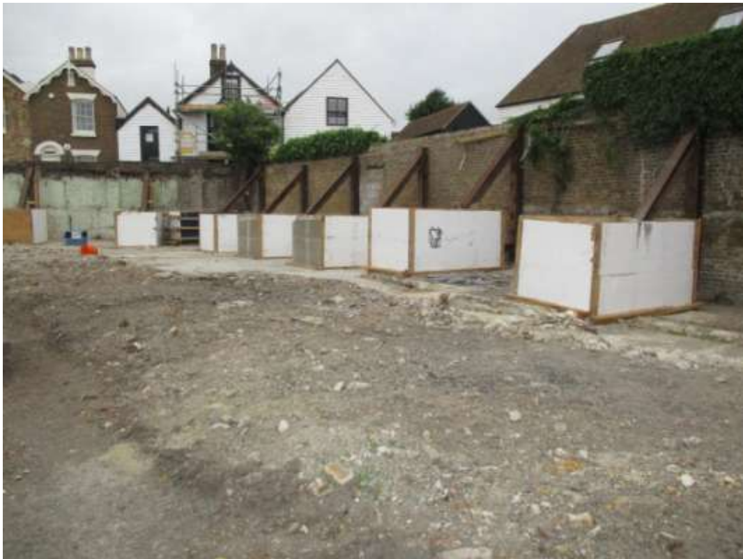
Plate 2. The substantial modern boxed-concrete wall supports supporting the eastern wall support
